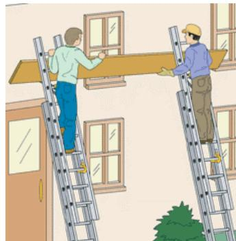
Place the plank into position onto the jacks. Make sure it is securely held by the jacks and extends at least 12 inches over at each end.
